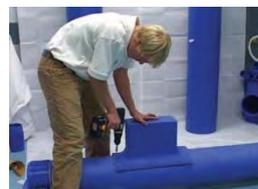
Secure both ends and drill screws
