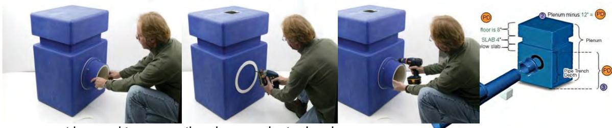
All screws must be used to ensure the plenum adapter has been sealed. The images below illustrate how to create and use a template marked area.
