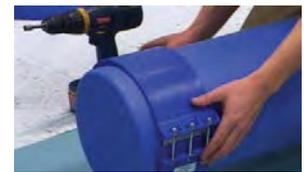
Slide clamp over gasket and tighten screws
